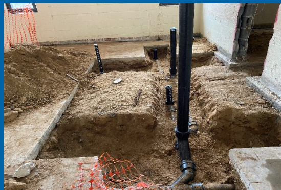
Trenching for Install of New Sanitary Pipes
