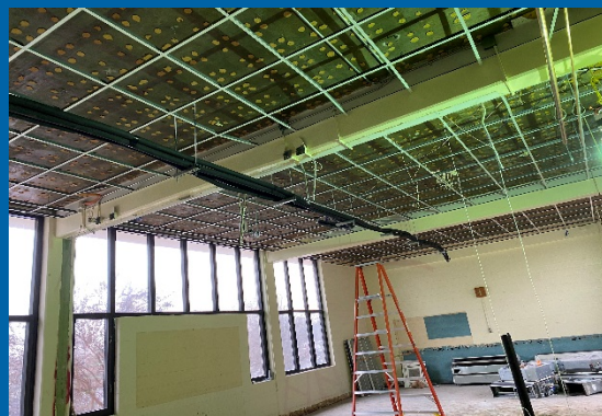
Removal of Mini Blinds and Reworking Ceiling Grid at 2010 for New Light Fixtures
